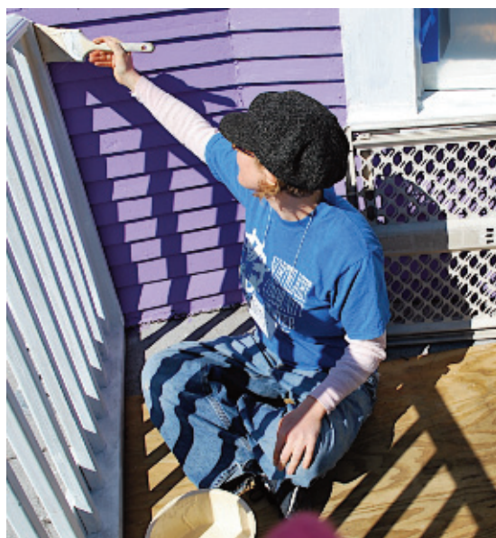
Painting a Katrina-damaged house in New Orleans.
