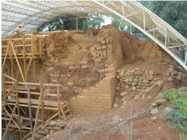
Restoration work begun on the northeastern gate tower
